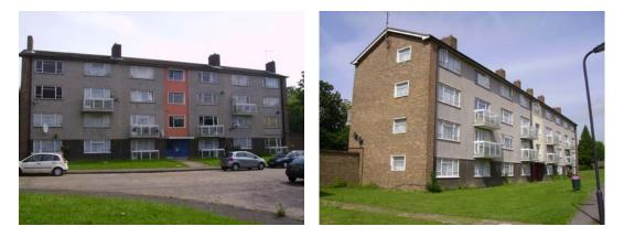
The Easiform system of building is a cast insitu concrete form of house construction developed by John Laing. The first house was built in 1919 and approximately 5,000 dwellings were completed during the inter-war years, most of which were erected in the mid 1920's. The Easiform system was reintroduced after the war in 1946 and was in production until the early 1970's providing a further 85,000 dwellings.
